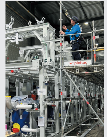
Operator performing an assembly operation on a hydrogen station
