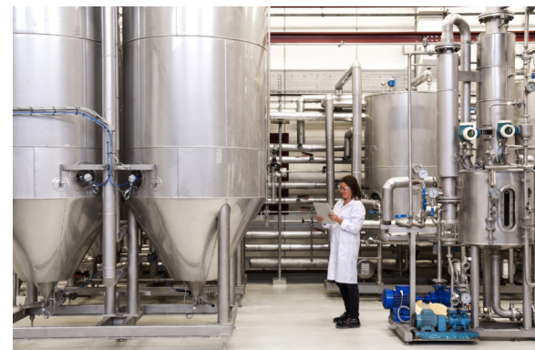
Boccard technician monitoring an installation
